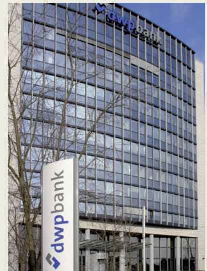
dwpbank's Düsseldorf offices
